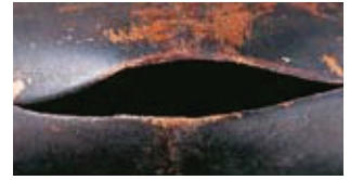
FREEZE RUPTURE Caused by low water flow in the evaporator.
