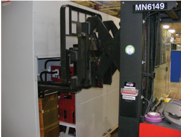
Figure 32. Inserting the CMC into the CMC cabinet
