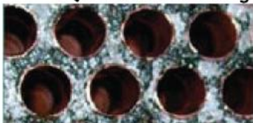
▽ Tube after cleaning
