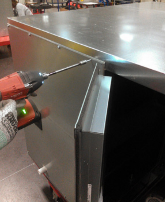
Figure 1. Remove roof panel
