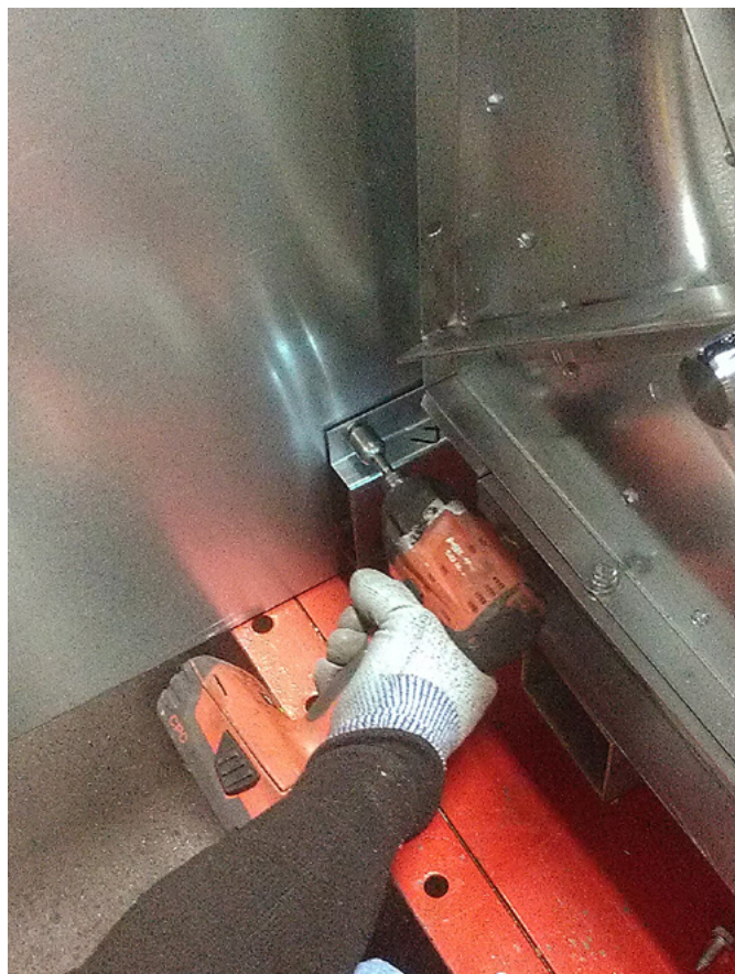
Figure 20. Support walls to prevent falling
