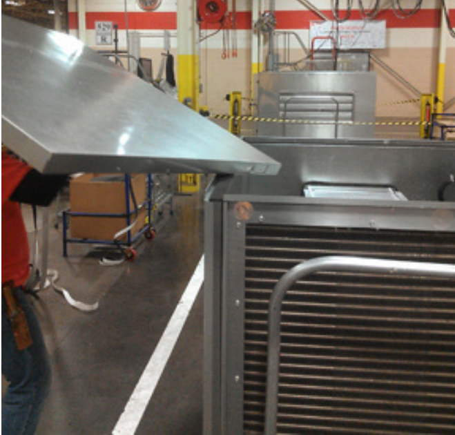
Figure 8. Lift the roof panel off
