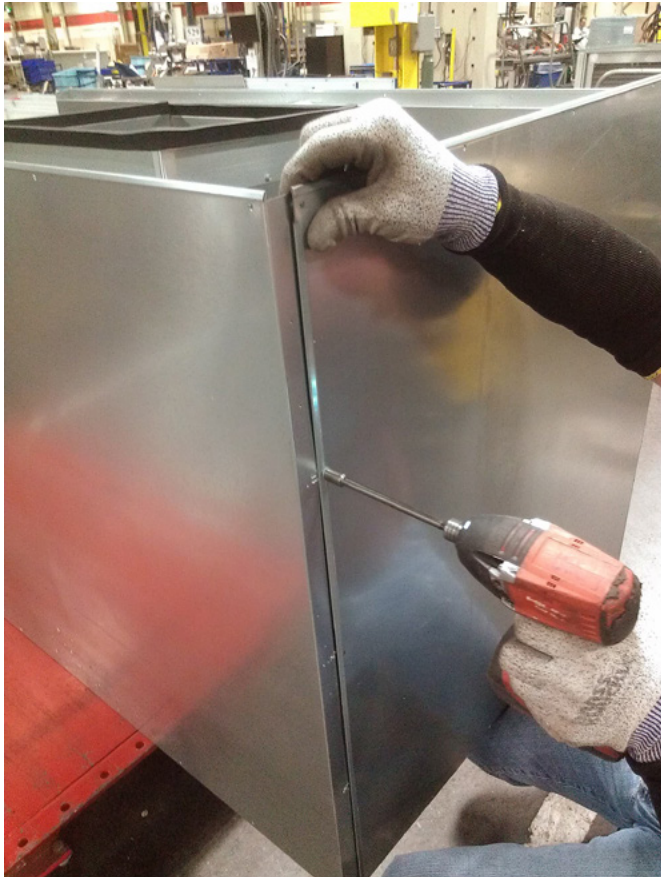
Figure 11. Remove the wall panels
