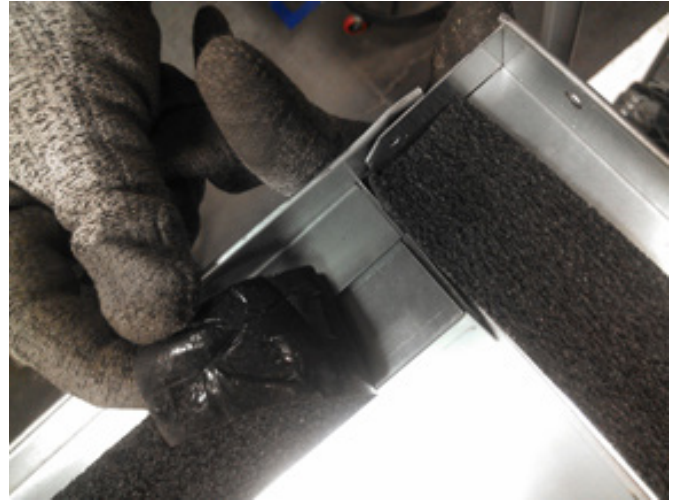
Figure 10. Gasket details at top corner
