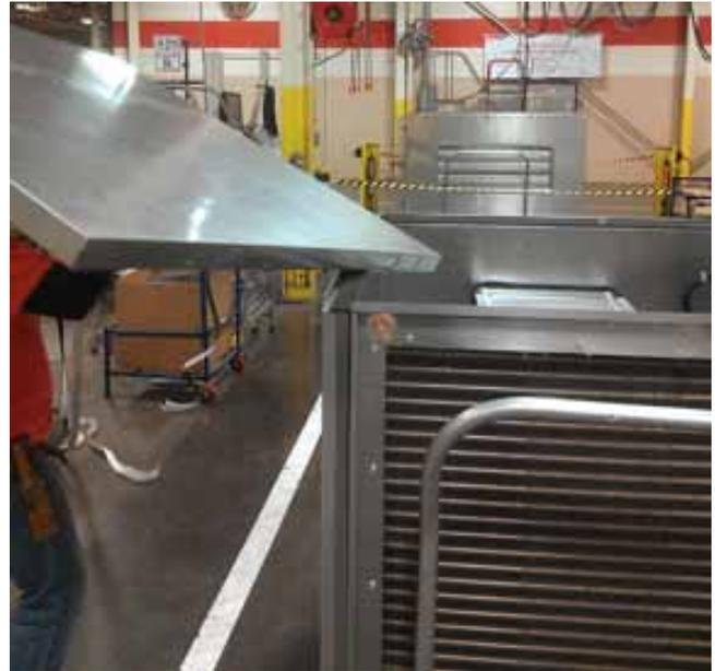
There is gasket along top of the unit at the COU panel and wall panels. The gasket should be in good condition to be reused, but if not, the gasket will need to be replaced. The door flange will have gasket along top and bottom as shown above and not on the top like wall and COU panels.
