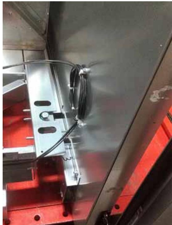
The walls and fan need to be supported when the ½-inch screws are removed.
