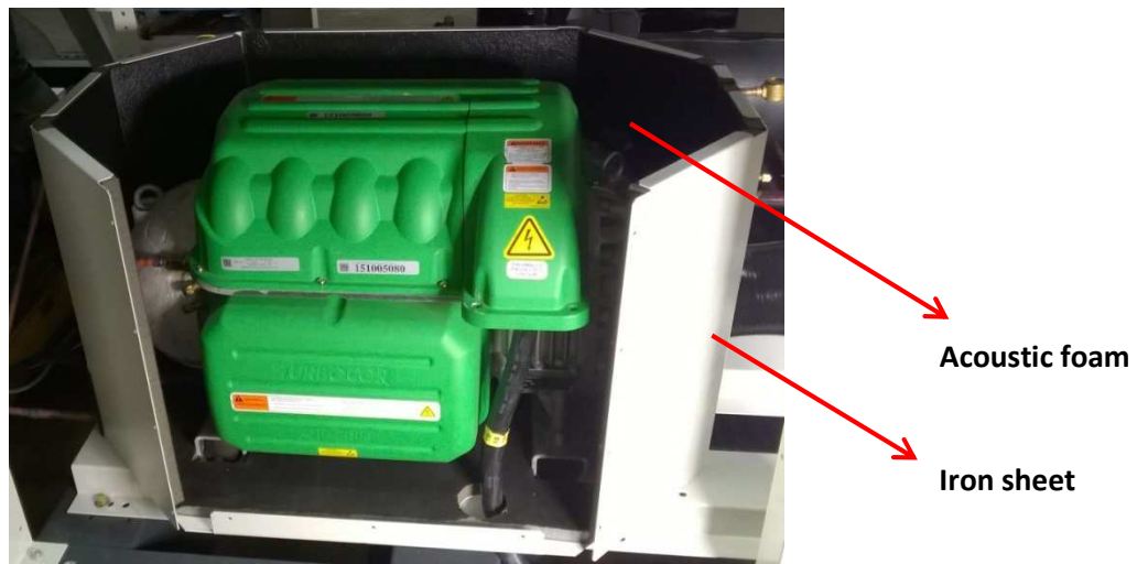
Illustration compressor insulation
