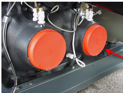
Illustration Evaporator water connection
