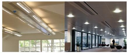
Returning to the same example, four 6-ft long active chilled beams are needed to offset the space sensible cooling load for this 1000 ft<sup>2</sup> office space (Figure 11). Notice how much ceiling area is covered with the beams.
