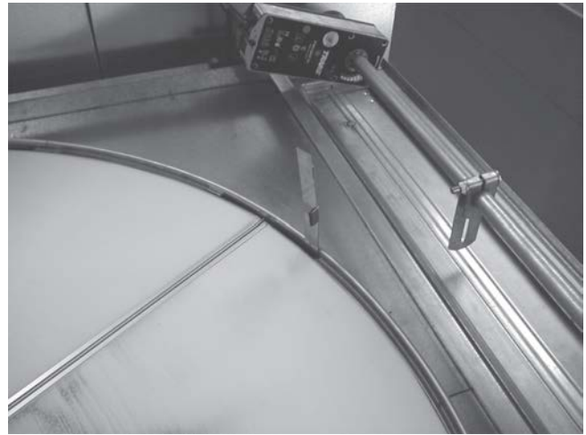
Figure 170. Completely fasten segment retainers
