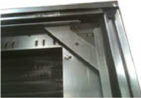
Figure 28. Coil structural gusset
