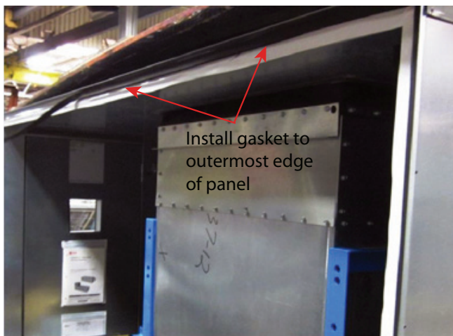
Figure 32. Install gasket to outermost edge of panel
