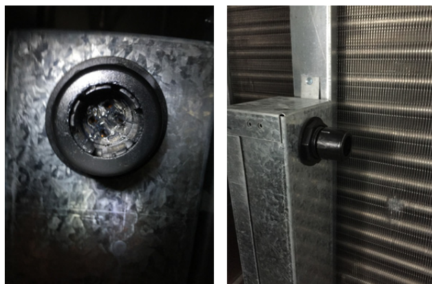
Figure 207. Plug pins into socket, then tighten compression nut
