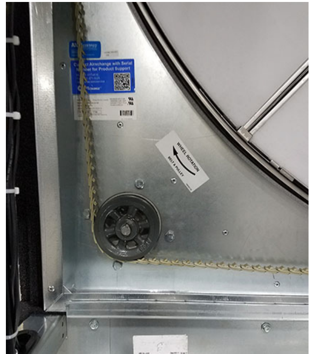
Figure 171. Confirm proper belt tracking on wheel rim
