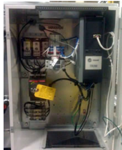
Figure 147. Externally mounted VFD
