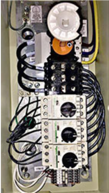
Figure 148. External motorized impeller control panel (MICP)
