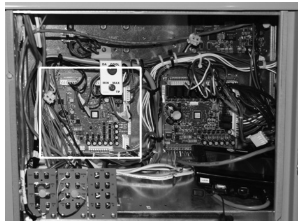
Figure 13. Precedent™ E Cabinet - RTOM board
