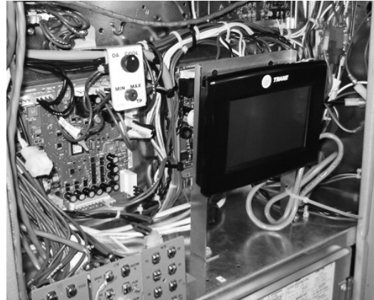
Figure 16. Precedent™ B Cabinet - TD-5 Human Interface
