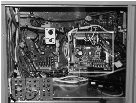
Figure 11. Precedent™ B Cabinet - RTRM board
