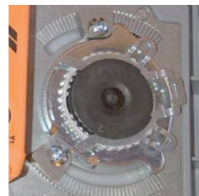
Figure 84. By-pass valve setting photo
